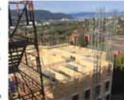
Shelter with no weather protection, Høvedskjøl, Nordland, Norway
