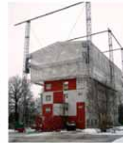
Example of climbing weather protection for sky construction with a high degree of prefabrication
